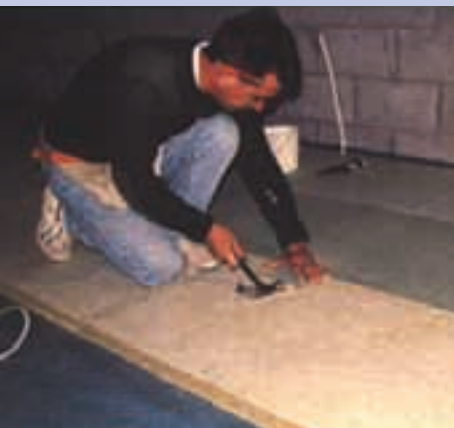
Chipboard being applied as a floating floor construction
