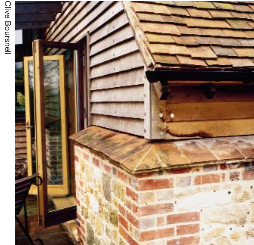
Figure 8 Built example using unseasoned oak cladding, by Gale and Snowden Architects
